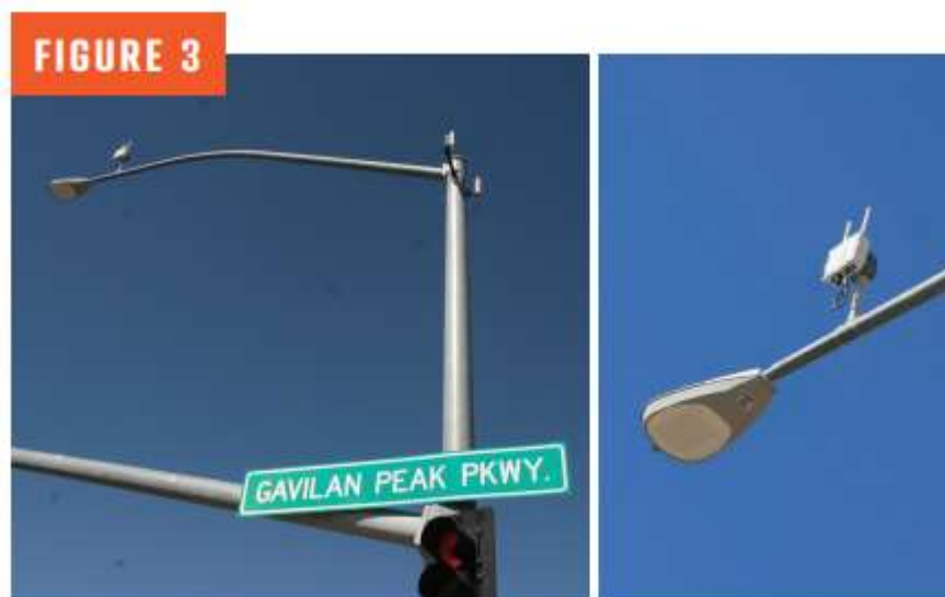
DSRC Radio Unit Installed on an Intersection Luminaire
